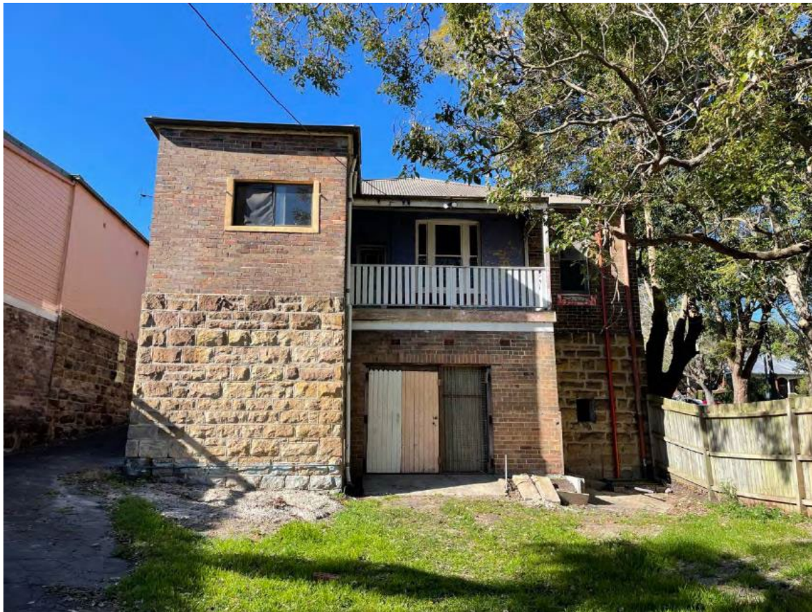
rear of existing dwelling on site - looking south-east
